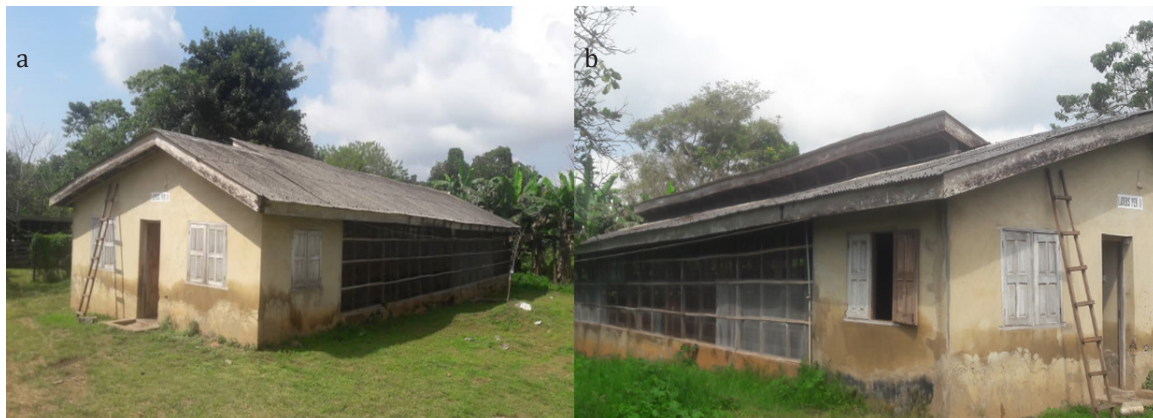
Figure 1. Naturally ventilated poultry building views (a) windward side and (b) leeward side.
